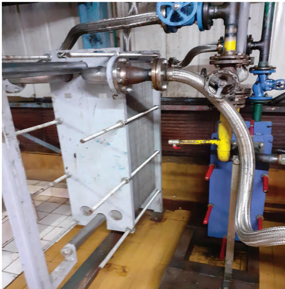
Slika 2. Razmenjivači toplote ulje-voda paralelno povezani Figure 2. Oil-water heat exchangers connected in parallel
